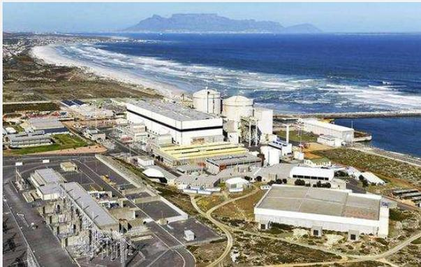
It has operated safely and efficiently for 30 years and has a further active life of about 20 years. Koeberg Power Station has a generating capacity of 1860 MW (sent-out). The 2 units are rated at 970 MW each.
